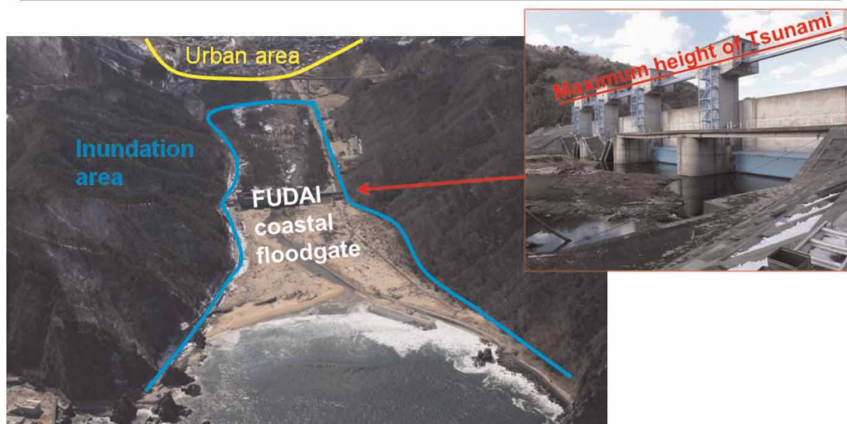
Fig. 6. An example of structural measures that provided protection against a tsunami that exceeded the defense-design capacity.
