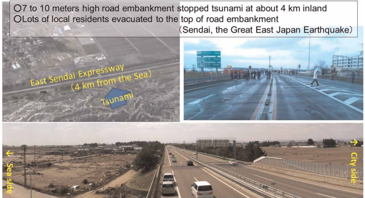
Fig. 3. An expressway functioned as a tsunami barrier and an evacuation site.
