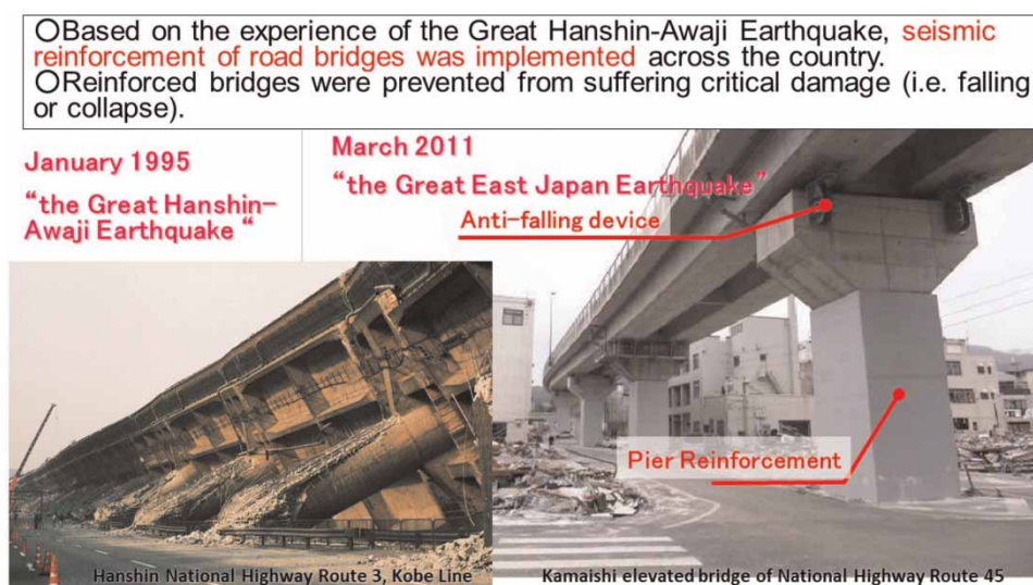
Fig. 1. Effect of seismic reinforcement of bridges after the Great Hanshin-Awaji Earthquake.
